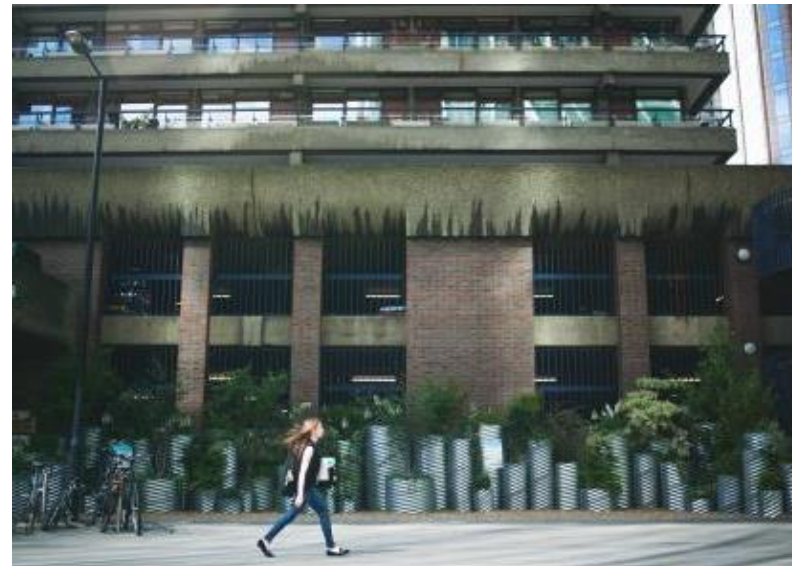
What the site looked like after installation
